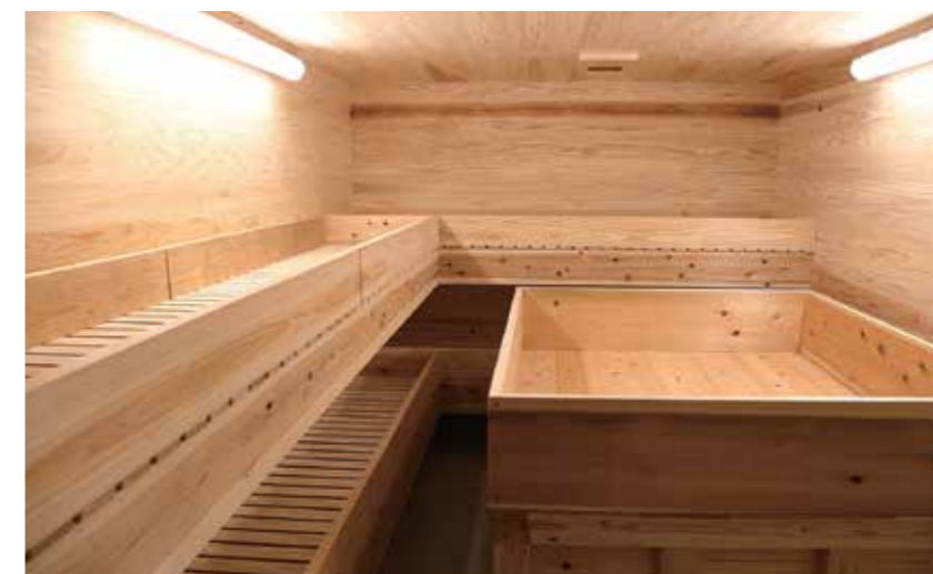
The interior of the new koji room is now visible from the outside. A double-layer of doors with a gap between them minimizes any temperature fluctuations inside the chamber.
